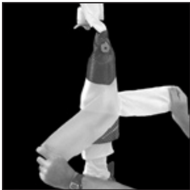
Ref.10 Apply Carbon Fabric Et Fiberglass Strip
